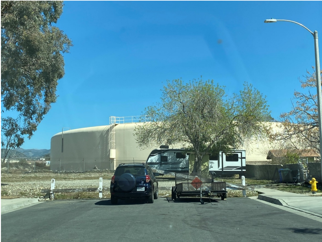
Photo 2 - View facing northwest, looking the West Valley Water District reservoir at the western end of W Via Bello Drive.
