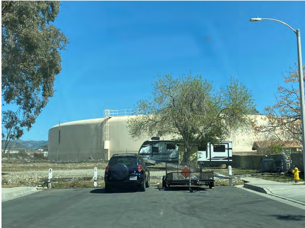
Photo 2 - View facing northwest, looking the West Valley Water District reservoir at the western end of W Via Bello Drive.
