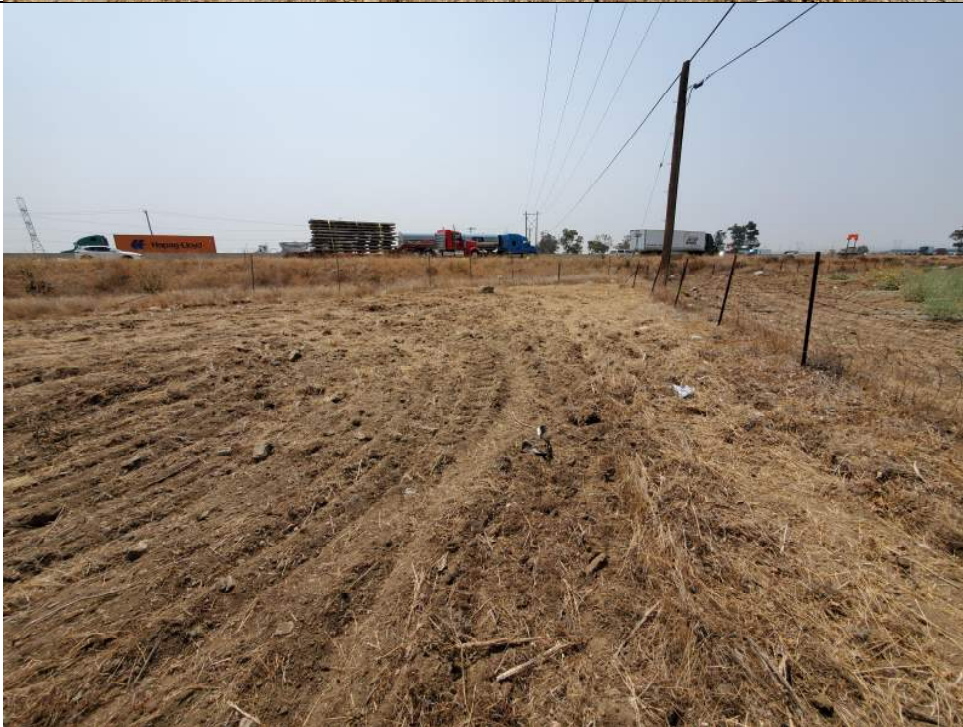
Photo 4. Approximate location of proposed jack and bore pit on north side of I-15.
