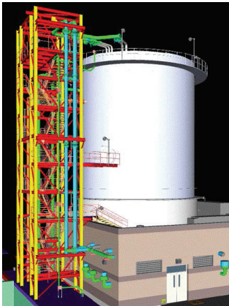
PCL produced a 3-D model of our recently completed PAR 1280 Project for Metro Wastewater Reclamation District.
