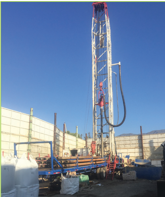
Borehole reaming for the Miragrاند Well
