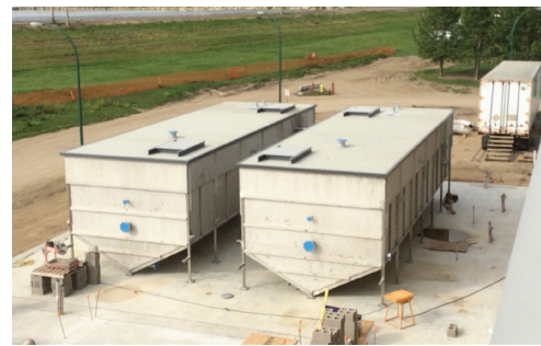
Packaged DAF Thickeners under construction, designed by Stantec.
