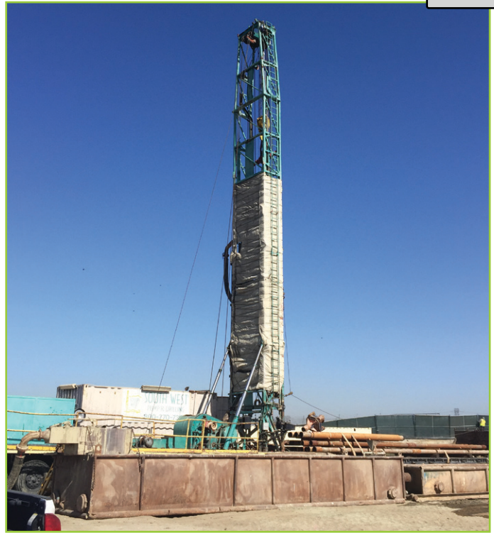
Pilot borehole drilling for CDA-II-12
