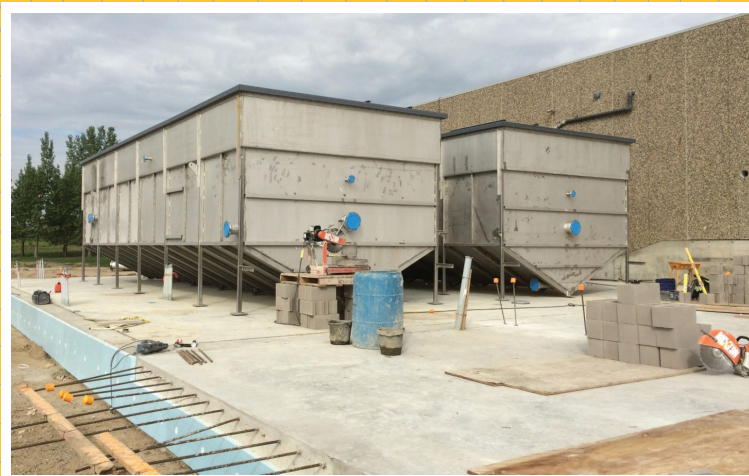
Packaged DAF Thickeners under construction, designed by Stantec.
