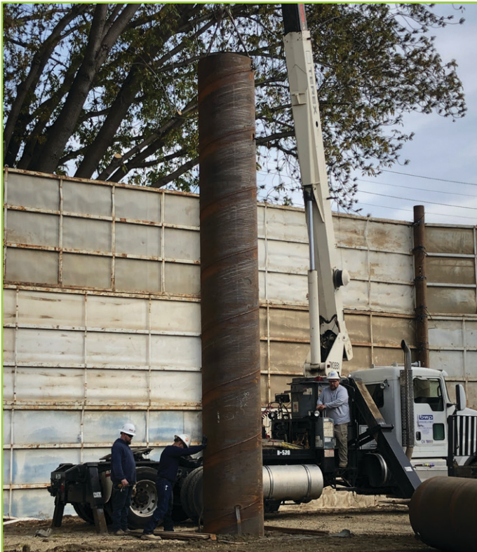
Installation of conductor.
