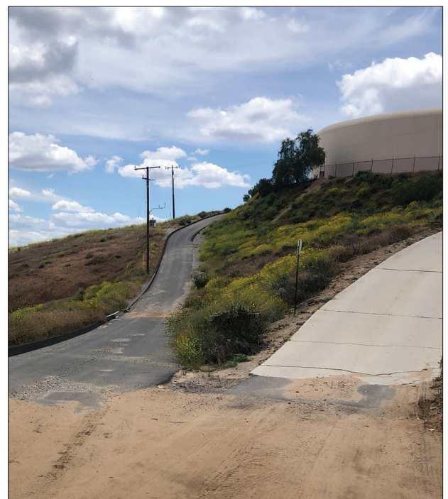
Looking south at Reservoir 3-1 at sediment on Alder
