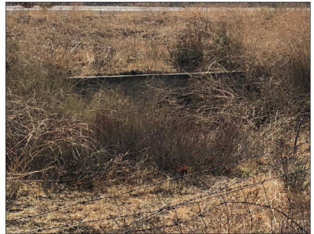
(Above) Cable Sign Along Lytle Creek Road (Below) Looking South at Existing Storm Drain Crossing I-15
