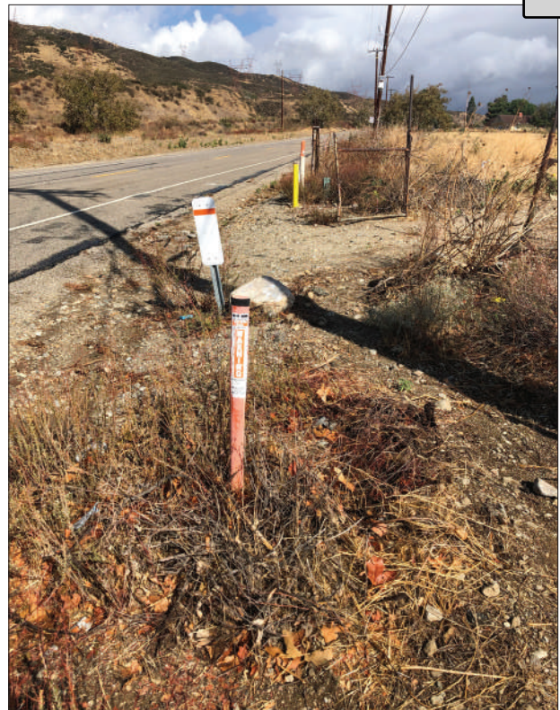
Looking North Along Lytle Creek - Buried FO Cable
