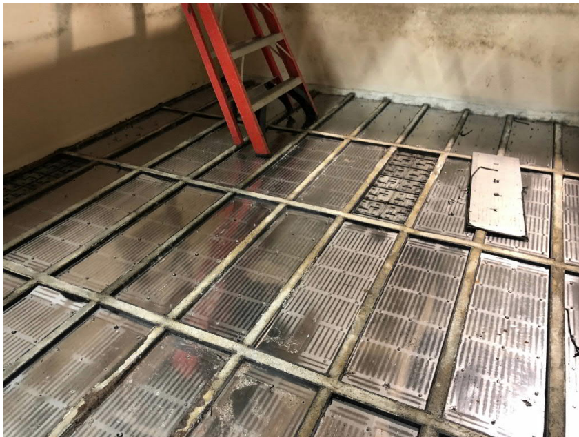
Grout between blocks appears to be in good condition
